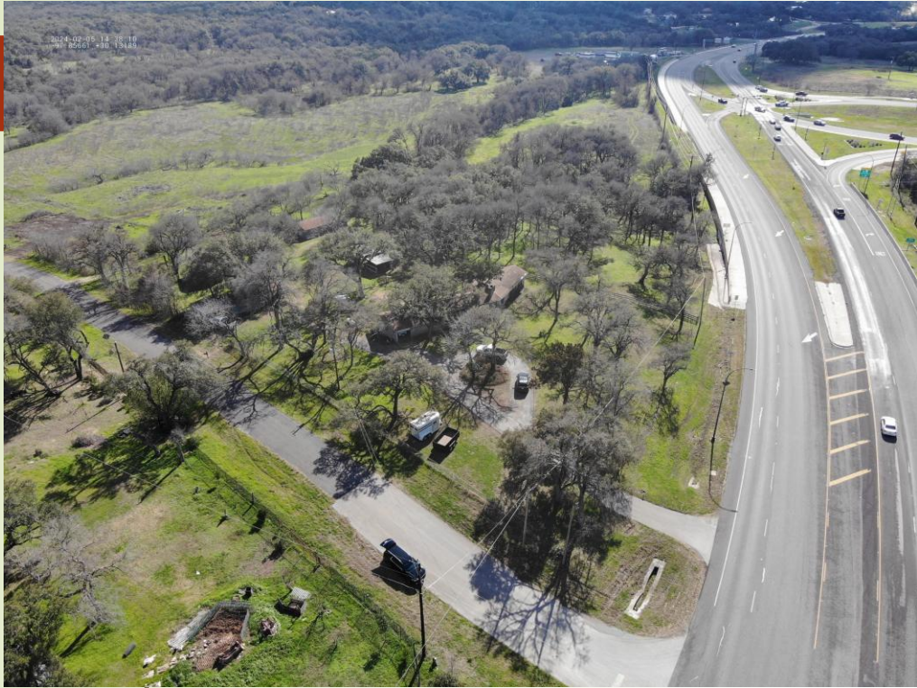
Big Valley Drive – 8 Multi Family Buildings – 303 Units
